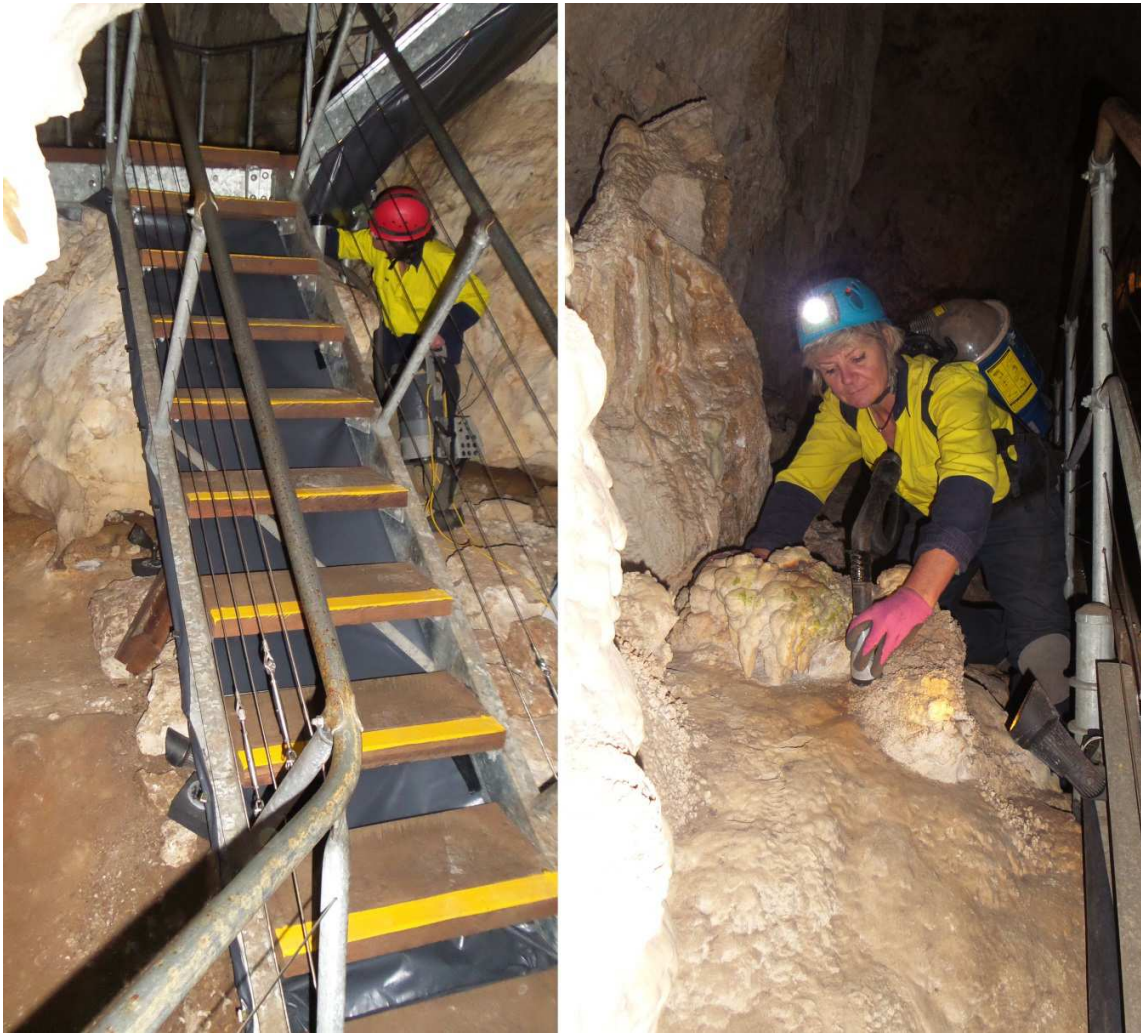
Figure 2: Dust diaper install and flowstone vacuum.
