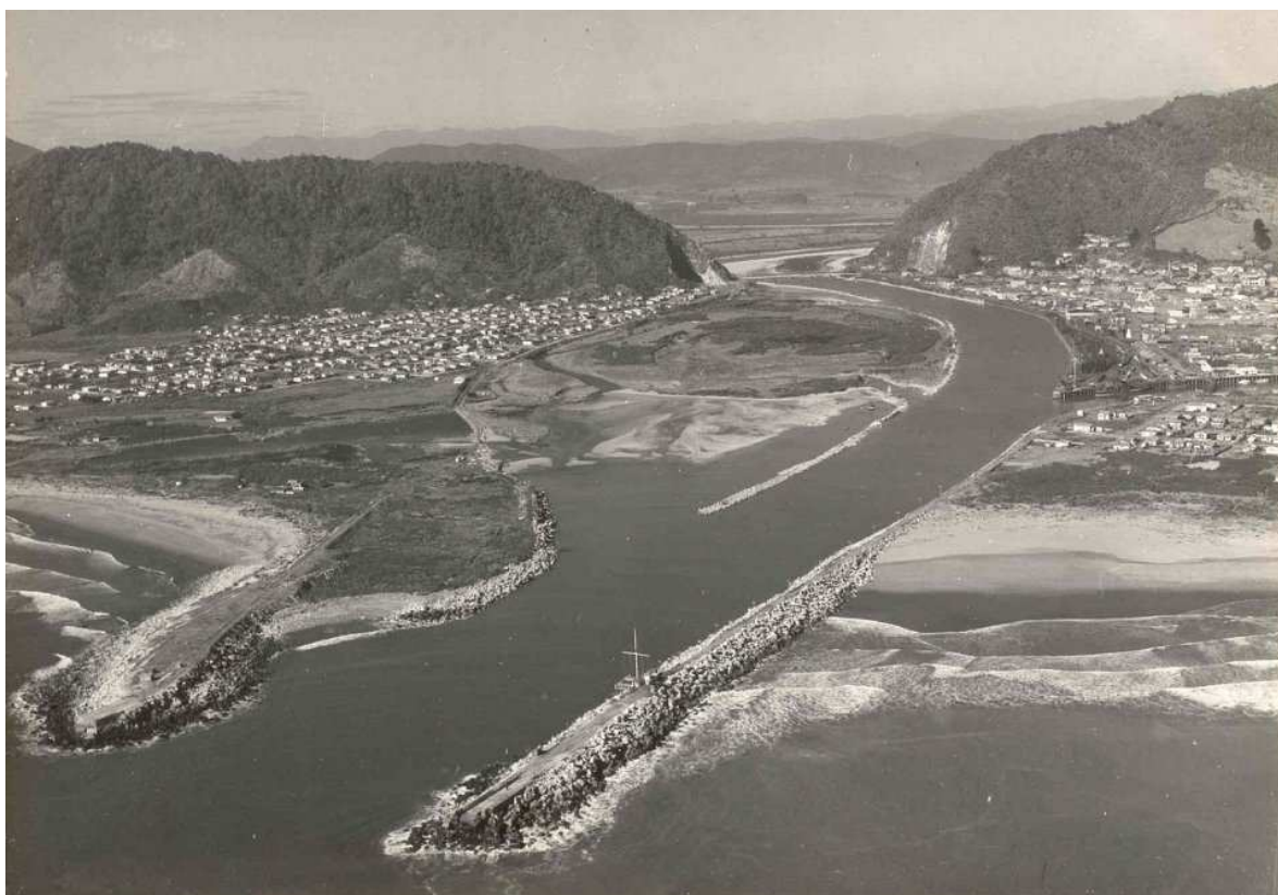
Figure 1: This 1950's White's Aviation photograph shows the north and south breakwaters, and a half tide wall along the Grey River. The Greymouth Gorge is in the back-ground with the obvious 'hole in the hill' on the left (north side) being the Cobden Quarry. Photo: History House Museum, Greymouth
