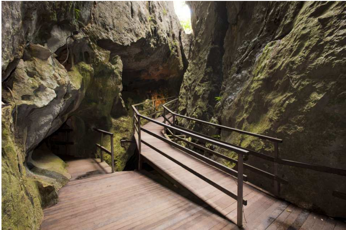
Wheelchair ramp constructed by Ken Augusteyn in 1992 with no visual impacts of timber stains.
