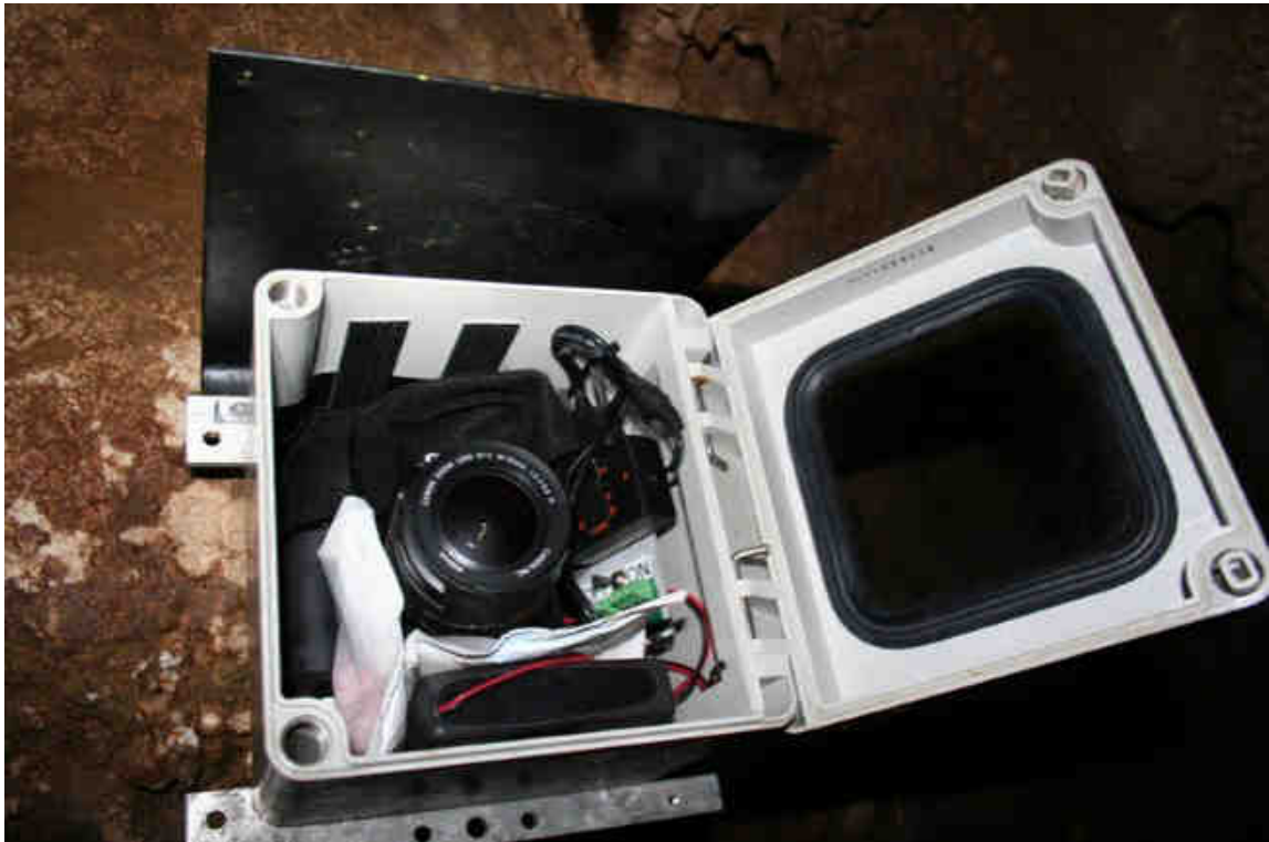
Figure 5. The Harbortronics time-lapse monitoring package installed in the Glowworm Grotto
