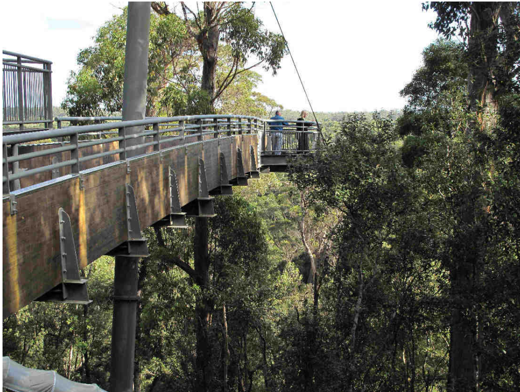
Figure 8 The Cantilever Viewing Platform.
