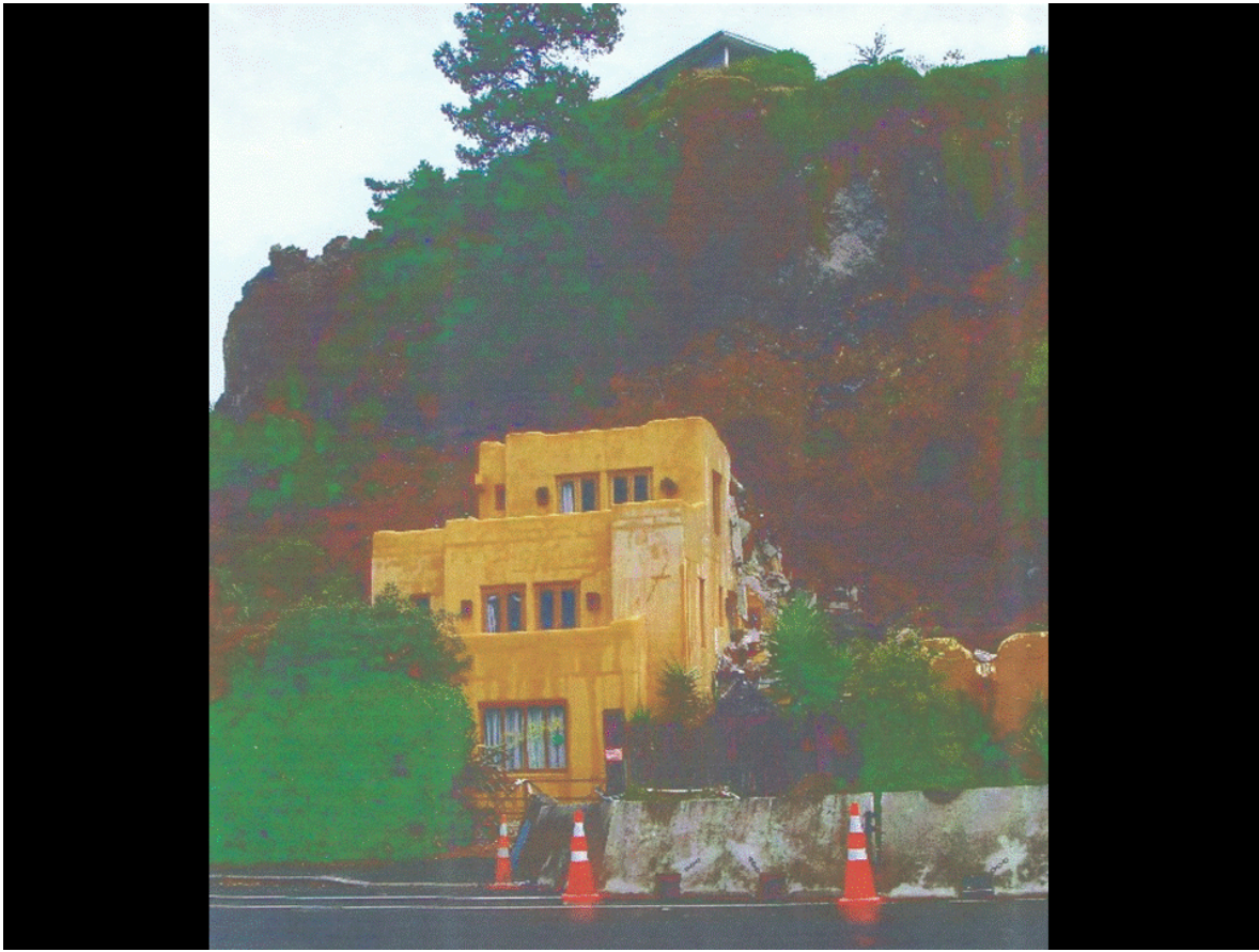
Figure 8: A house built over a cave is tottering over the edge waiting for an aftershock to collapse it on to the road below.
