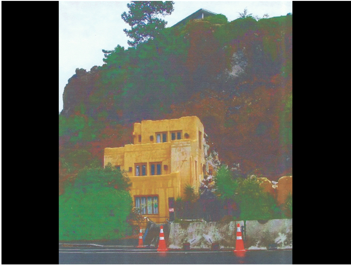
Figure 8: A house built over a cave is tottering over the edge waiting for an aftershock to collapse it on to the road below.
