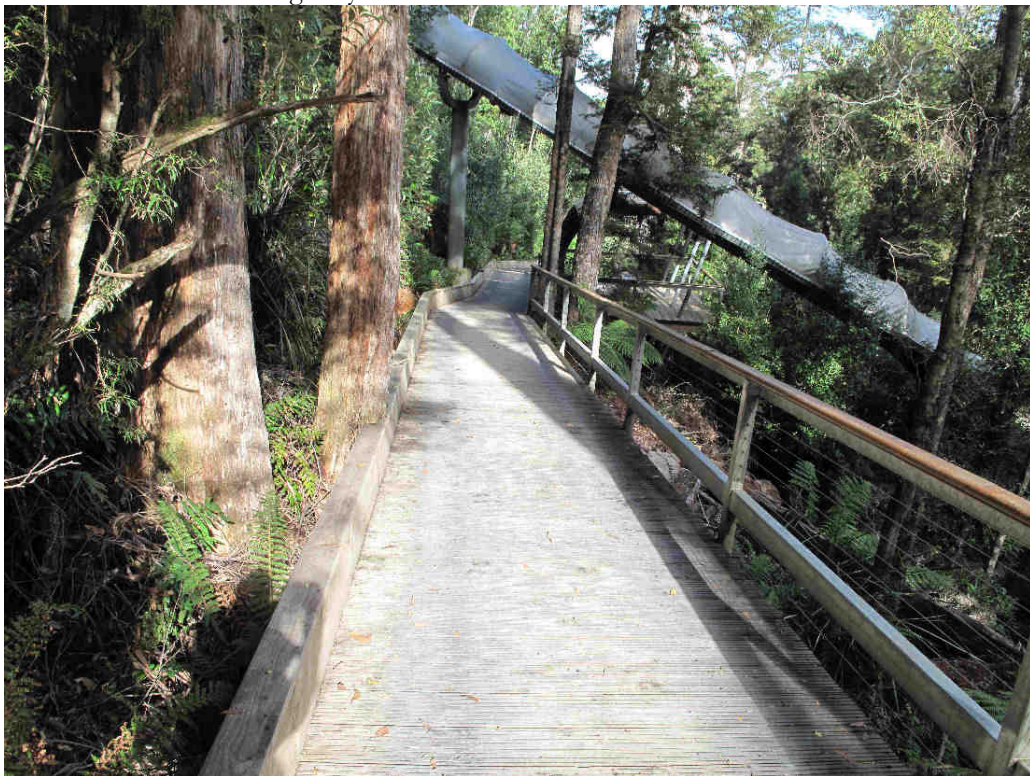
Figure 5. Use of boardwalk to minimise erosion on sides of sinkhole.
