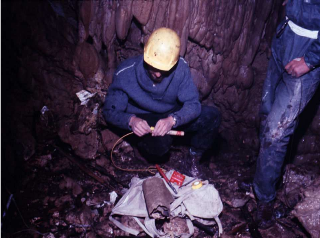
Photo: TCC Northern Branch's first attempt to blast through the entrance pitch of Execution Pot, Mole Creek, in May 1966. This image - Fusing the gelignite.
