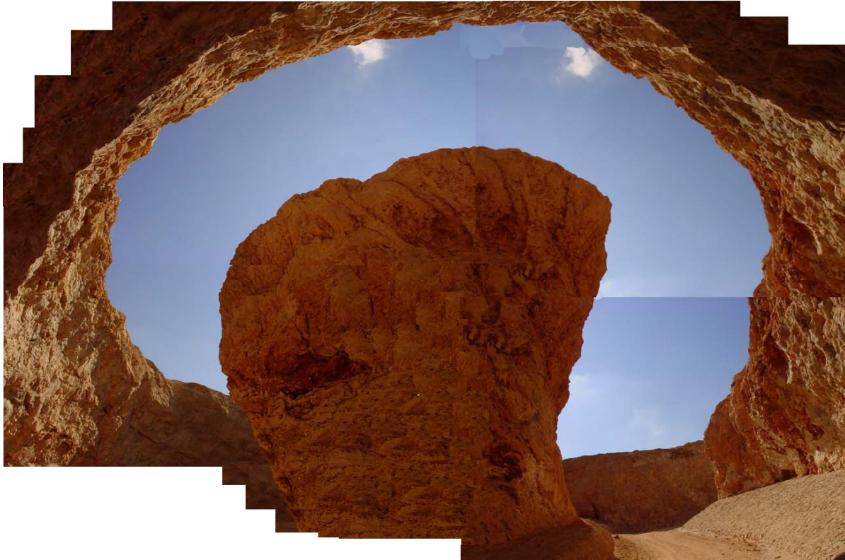
Fig. 4. Photo-montage of Sannur Quarry, looking up from the quarry floor. The faces overhang all around, extending out as far as 9 m in places. The access road comes from the right, leading down to the floor.
