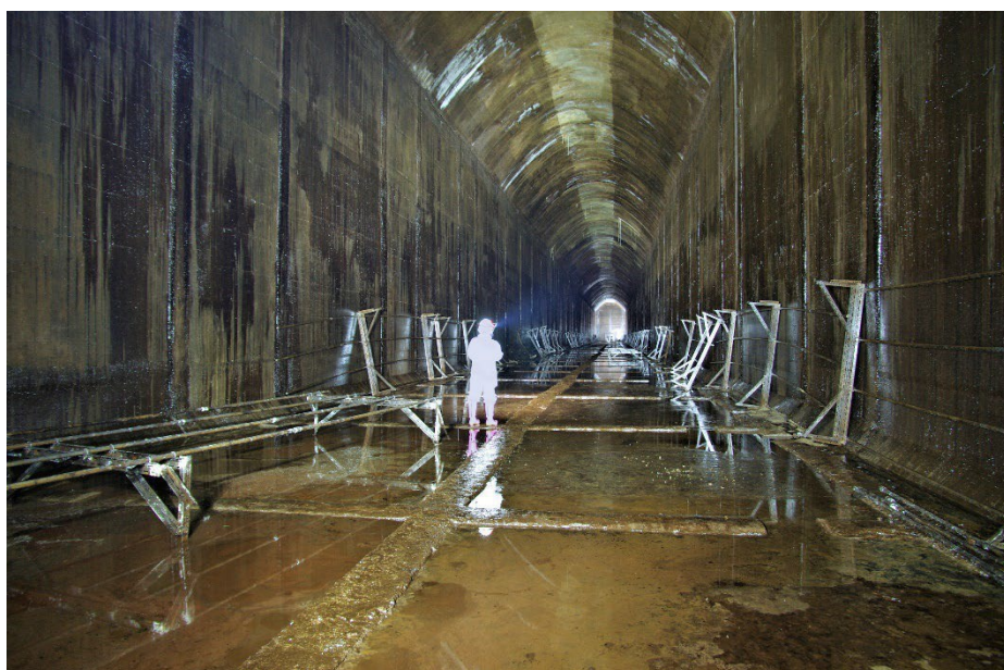
Figure 7: Interior of Tank 1, one of five identical tanks, each 237m long
