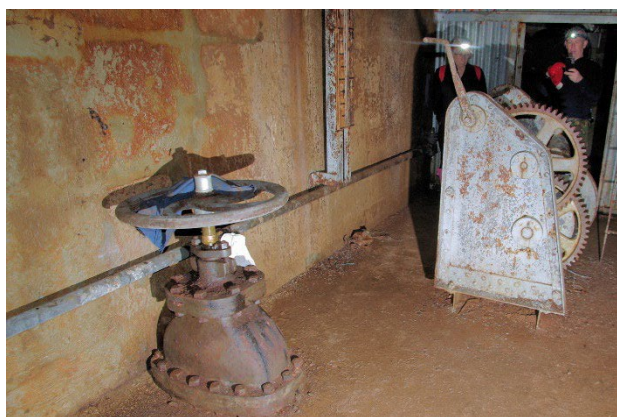
Figure 10: Hand operated valve and winching equipment for controlling oil flow from the tank (left)
