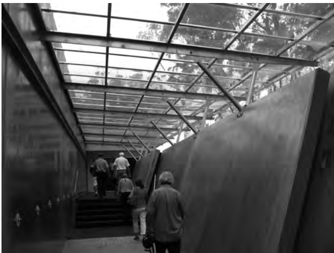
New access way connecting the new visitor center to the cave.
