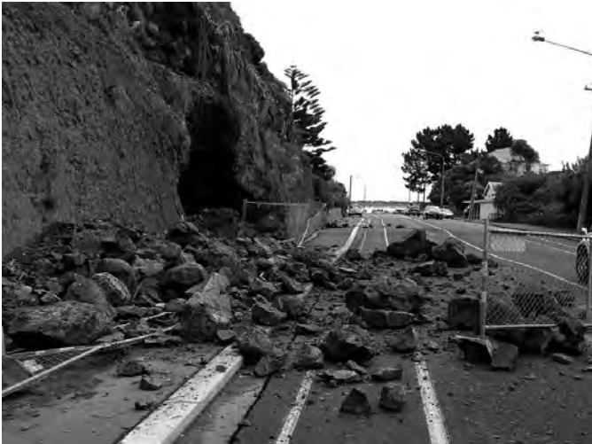
Moa Cave damage
