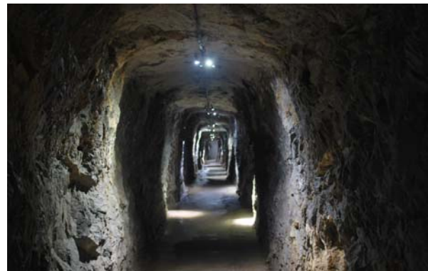
New LED lighting in the Binoomea Cut at Jenolan. Photo: David Rowling.
