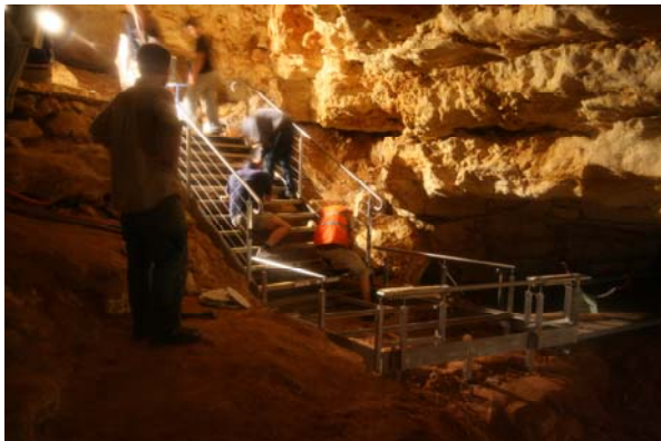
The new Fossil Site Viewing Platform under construction, Victoria Fossil Cave
