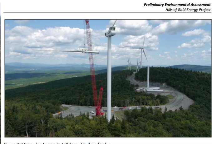
Figure 2-7 Example of crane installation of turbine blades
