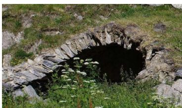
Perhaps the remains of a cellar but now used as a makeshift toilet!
