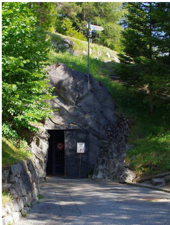
The entrance to the underground artillery fortress at Champex, Switzerland
