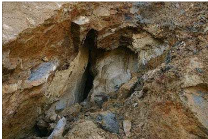
The cave in Tiropahi Limestone which was exposed during roadworks to re-align the highway at Pahuatane in 2009. The works were stopped thanks to due diligence by locals and West Coast cavers. Photo: F McDonald, Limestone Creek
