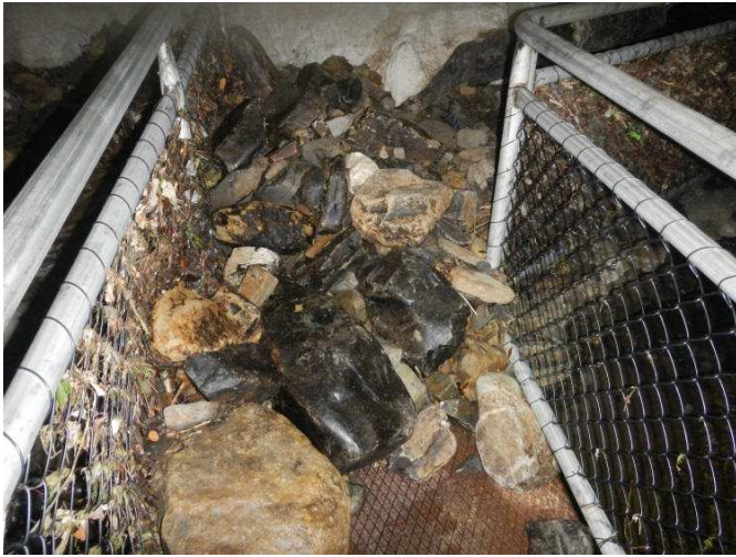
Bouldery debris deposited by floodwater on tourist path in Marakoopa Cave.
