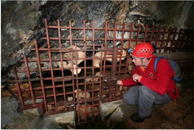
Ranger Dan Bowden inspecting the cave gate at Croesus Cave. Note boulders lifted by floodwater and pinned between the gate and cave entrance.
