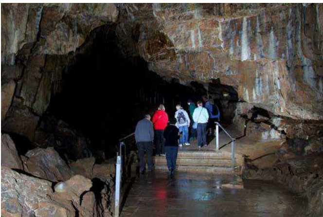
New stainless steel handrails, with steel posts, in Poole's Cavern. Photo: John Brush
