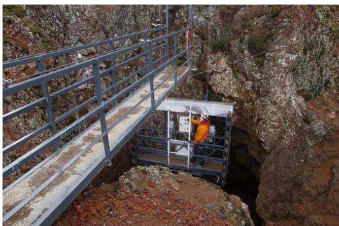
View of the approach walkway and lift platform for the Inside The Volcano descent. The wheels on the side of the platform are to keep it clear of the walls in a narrow part of the shaft.
