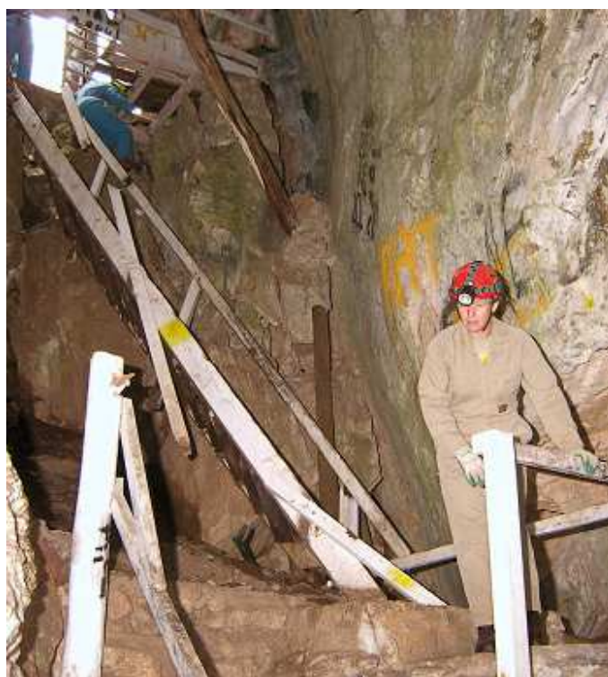
The remains of the fire-damaged entry stairs just prior to their removal in February 2005
