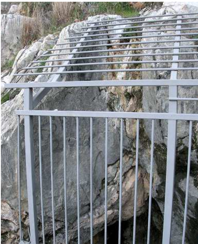
The new (2007) entrance was not 'bat-friendly' or vandalism resistant. Subsequent modifications were of limited success in overcoming these basic design flaws.
