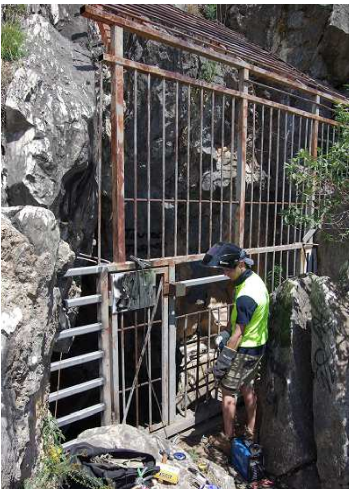
Above: The first day of work in January 2019 to replace vertical rods with horizontal square-section tube
