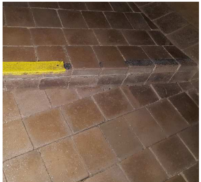
One of the missing stair tread safety strips
