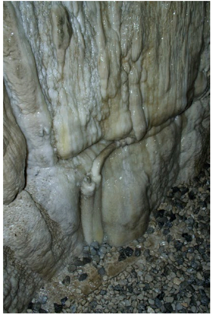
Calcite encrusted electrical cable Photo: John Brush
