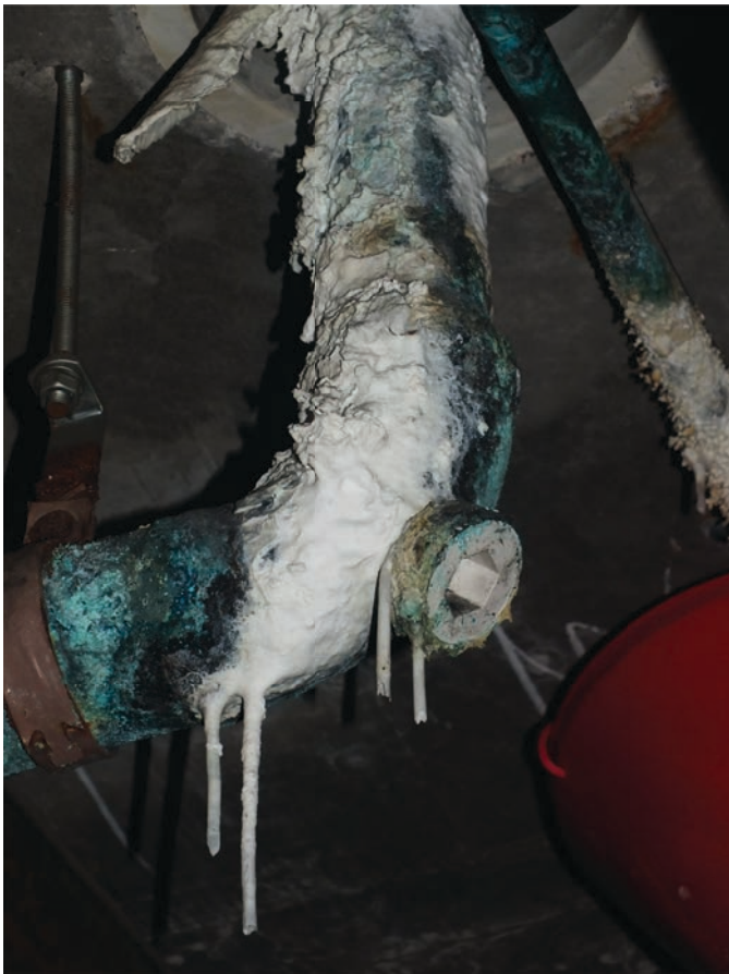
Examples of Calthemite straws in an underground carpark
