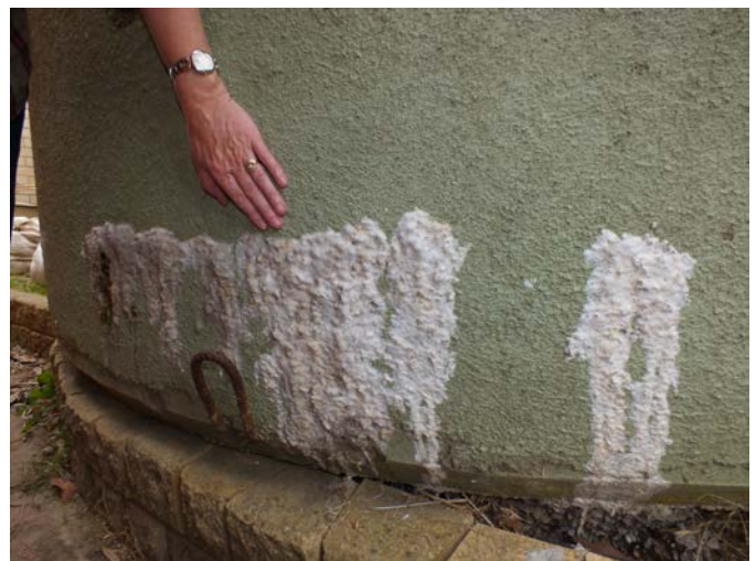
Example of Calthemite flowstone on concrete water tank
