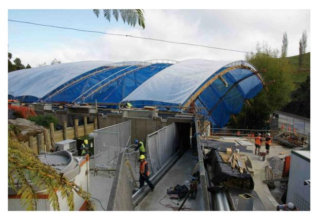
The concept for the structure was based on a hinaki (traditional Maori fishing trap) with the main frames supporting the Efte (Teflon) pillows canopy, constructed of large curved laminated timber beams representing the woven pattern of the fishing trap. This design channelled the visitors through to the cave entrance. The
